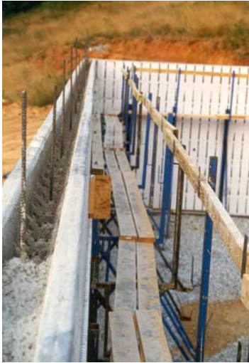
Figure 1. Sandwich wall under construction
